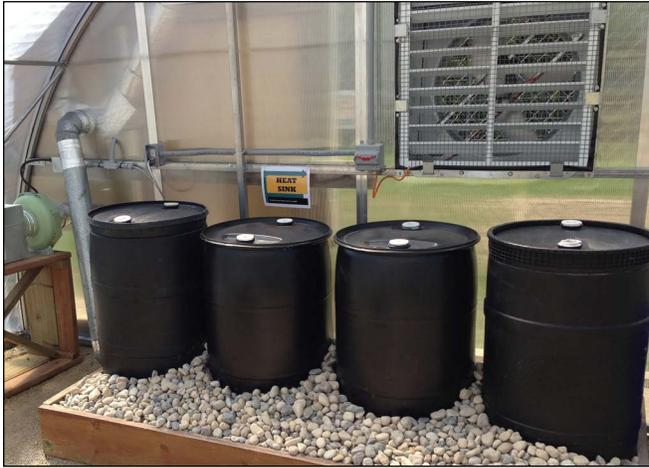
Old plastic barrels are used to make a heat sink in the LES Grow to Give Greenhouse.
