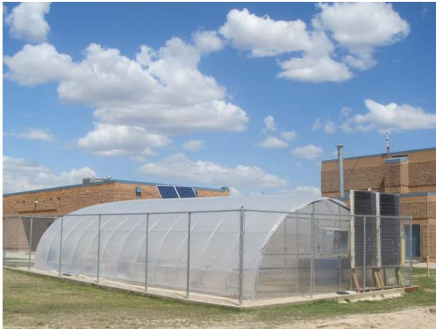
The pop can solar heaters at the back of the Grow to Give Greenhouse at LES collect heat during the day and pump heat into the heat sink units so that temperatures in the greenhouse are moderated during the cool nights of the growing season.
